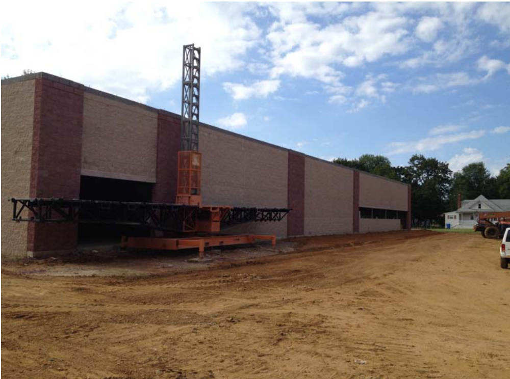
Clayton Shopping Center Clayton, NJ (Completed 2015)
