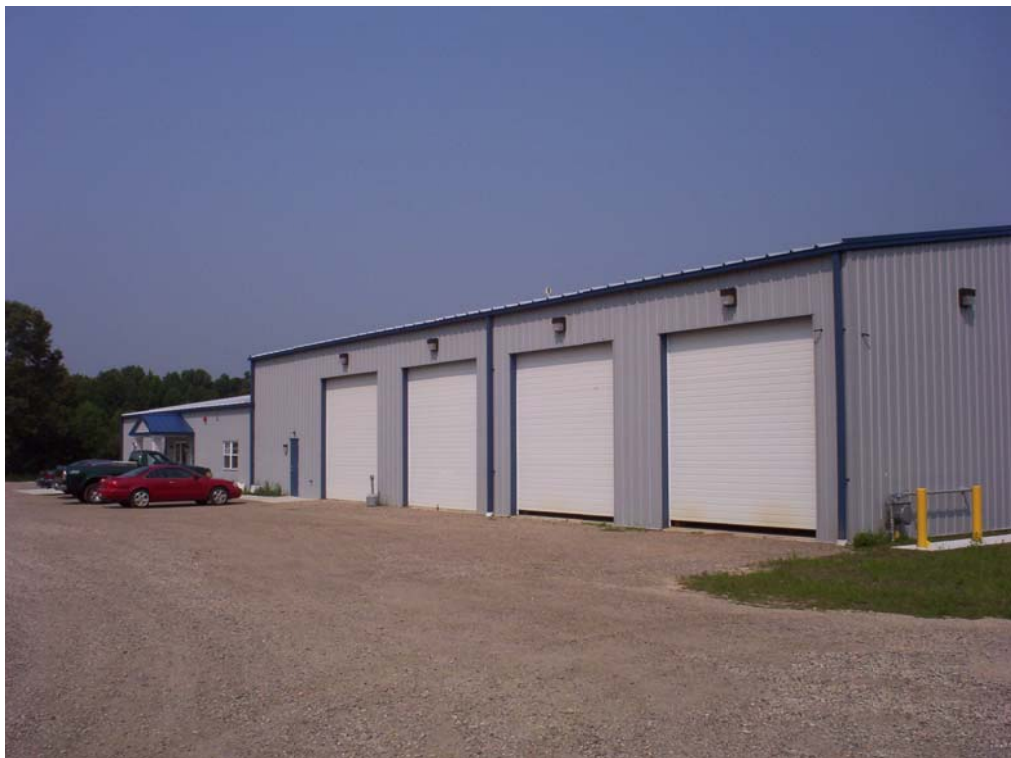
Uni-Tech Drilling Co., Inc. Franklinville, NJ 08322
