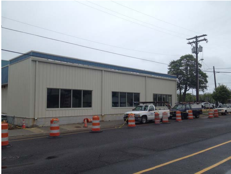
Holley Beach Volunteer Fire Station - Addition Wildwood, NJ (Completed 2015)
