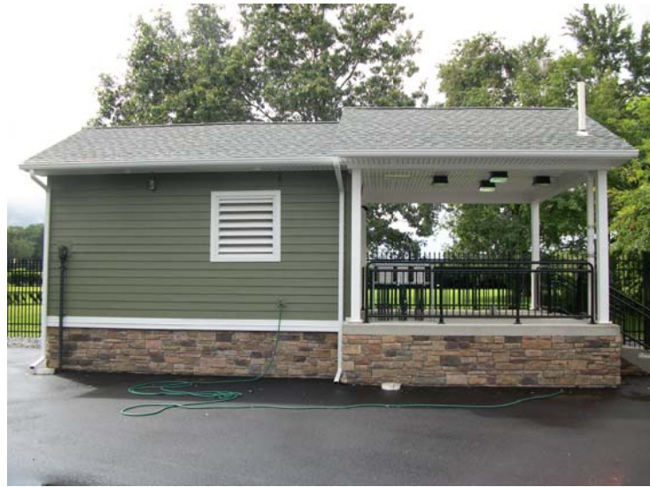
Hamilton Twp. MUA - Main Street Pump Station Mays Landing, NJ
