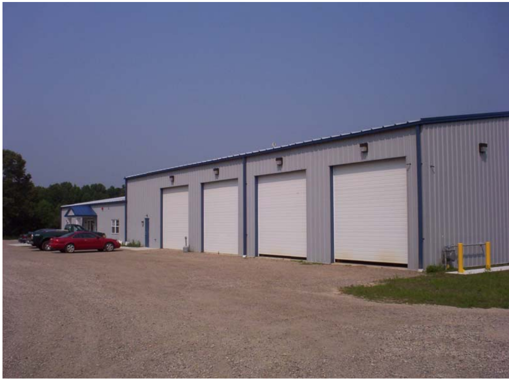
Uni-Tech Drilling Co., Inc. Franklinville, NJ 08322
