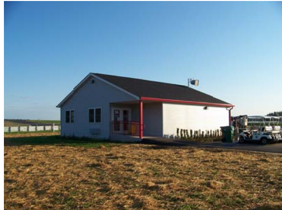
Medical Building - NJMP Millville, NJ
