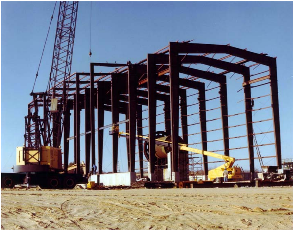
Unimen Dividing Creek, NJ
